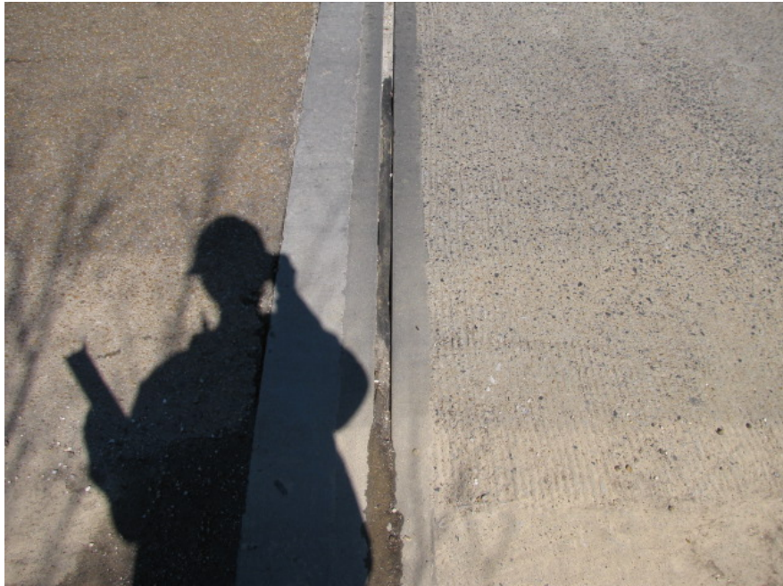
SPAN 1 JOINT MATERIAL PEELING(TYPICAL SPAN 5 JOINT)
